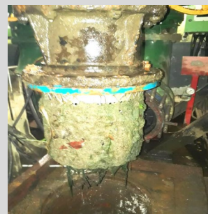
Unclogging of raw water pumps
