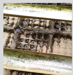
Sand filter refurbishment
